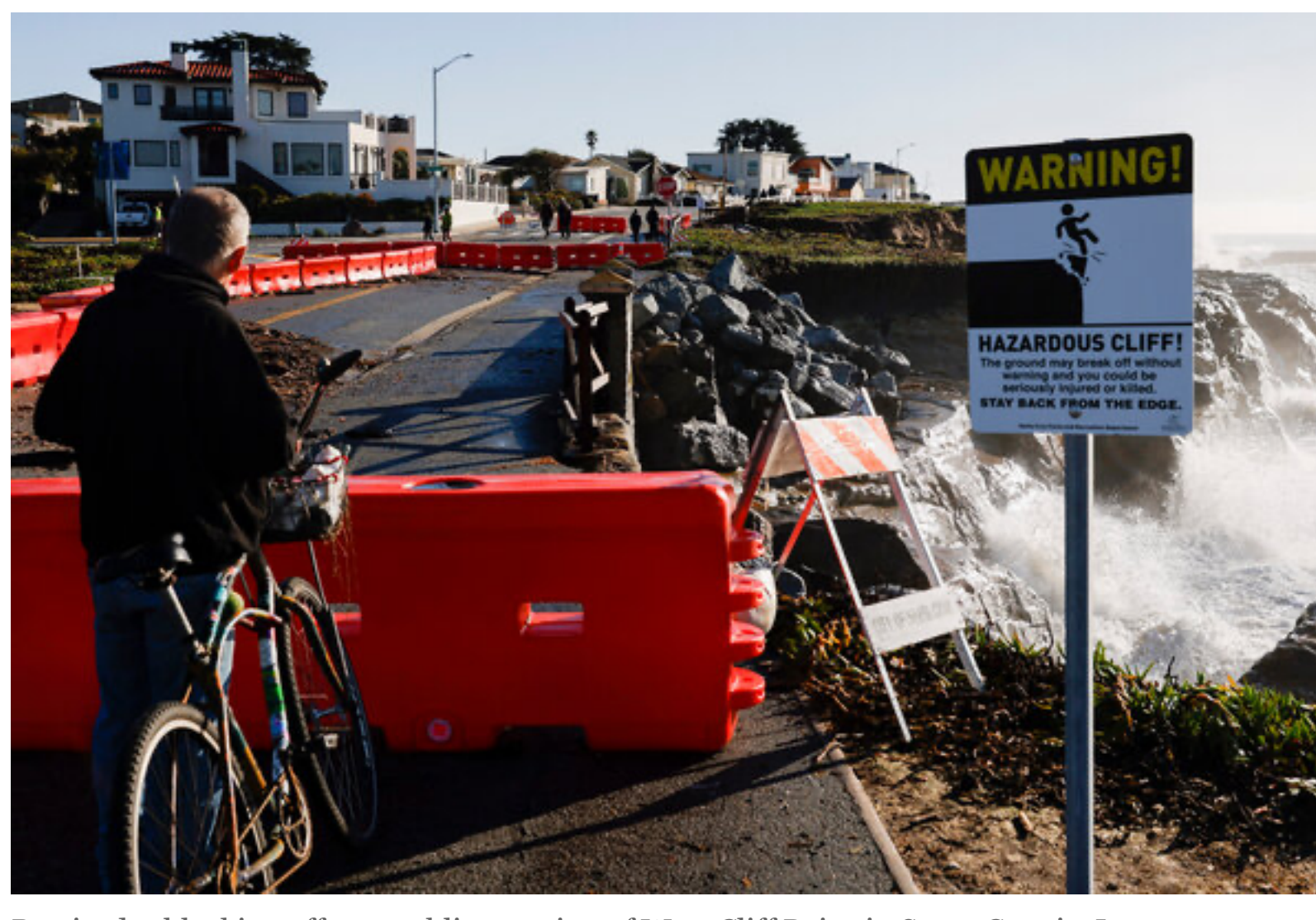
Barricades blocking off a crumbling section of West Cliff Drive in Santa Cruz in January. Jessica Christian/San Francisco Chronicle via Associated Press
